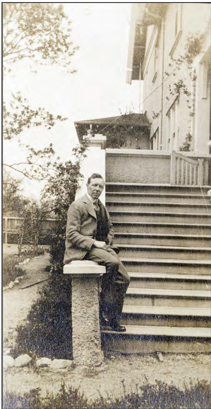
Fig. 11: Archival photograph showing the side staircase and back entrance to 960 Foul Bay Road. (Source: Uno Langman Collection UBC Robert Sinclair Album, 1-0053546.0010)
