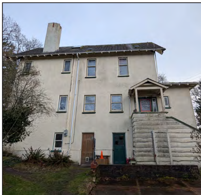
Fig. 17: Current view of the North elevation, 2025. (Source: Cummer)
