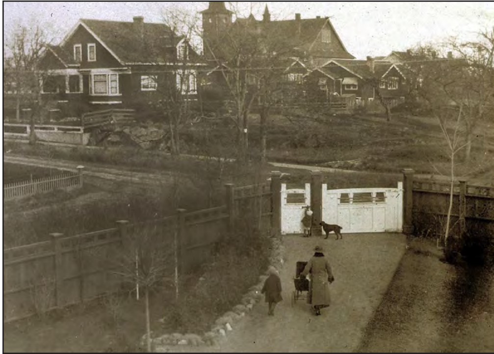
Fig. 12: Archival photograph showing the view from 960 Foul Bay Road, illustrating the former look of the landscaping and fencing. (Source: Uno Langman Collection UBC Robert Sinclair Album, 1-0053546.0193)
