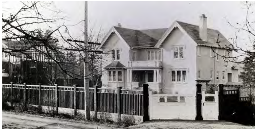
Picture of original fence along Foul Bay Road
