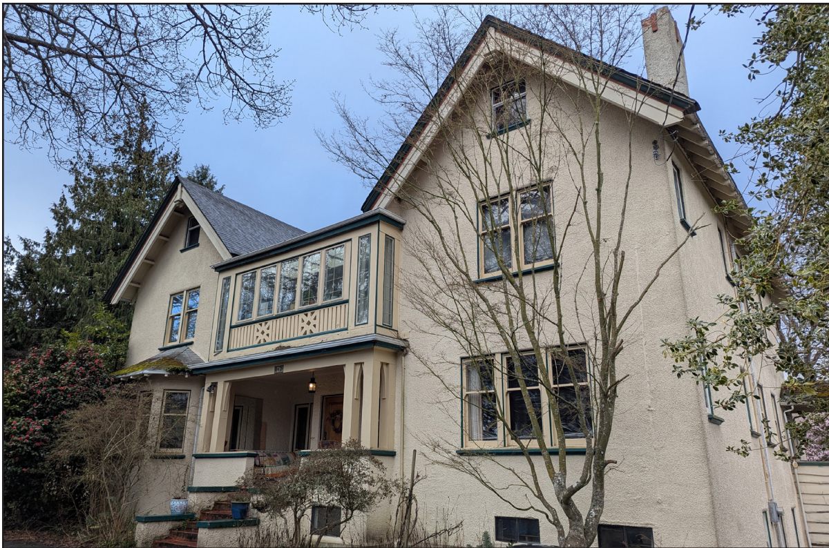
Fig. 2: Front view of 960 Foul Bay Road, 2025. (Source: Cummer)
