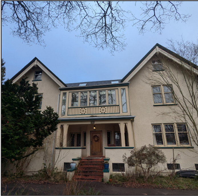
Fig. 14: Current view of the front elevation, 2025. (Source: Cummer)
