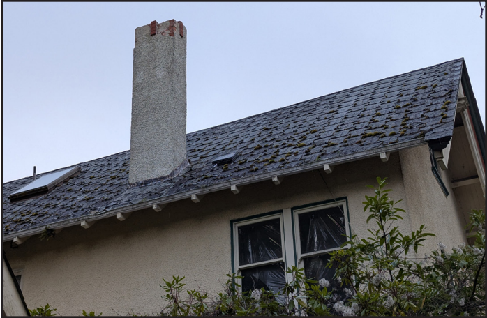
Figs. 23 and 24: Views of the northern side of the roof (above) and the southern side of the roof (below), 2025. (Sources: Cummer)
