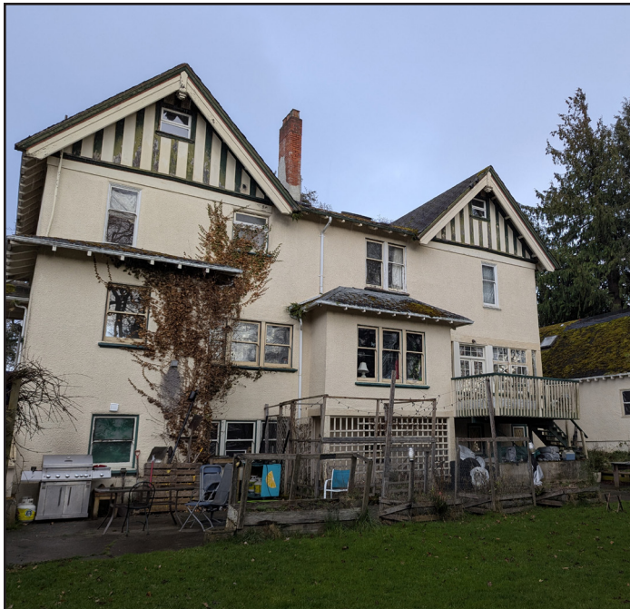
Fig. 16: Current view of the rear elevation, 2025. Note the later addition garage structure on the right, to the south. (Source: Cummer)
