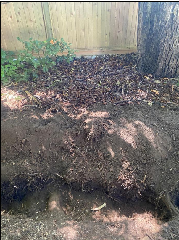
Photographs 6-9: Exploratory excavation within the CRZ of #987 encountered 1x >10cm Ø root at ~30cm south of the proposed "Building C" corner ( above ), 1x >10cm Ø root at ~4m south of the corner ( below ), a cluster of roots <5cm Ø and 1x 4cm Ø root ( upper and lower left ) at ~2-3m from the corner.
