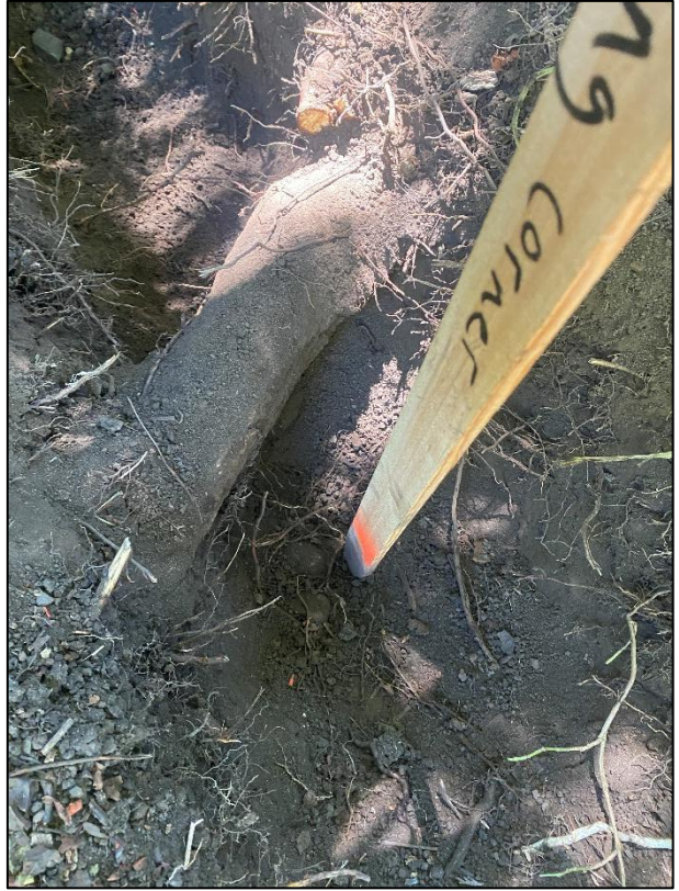
Photographs 6-9: Exploratory excavation within the CRZ of #987 encountered 1x >10cm Ø root at ~30cm south of the proposed "Building C" corner ( above ), 1x >10cm Ø root at ~4m south of the corner ( below ), a cluster of roots <5cm Ø and 1x 4cm Ø root ( upper and lower left ) at ~2-3m from the corner.
