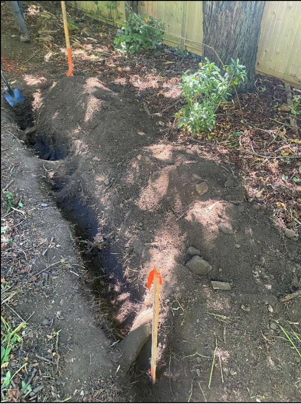
Photographs 6-9: Exploratory excavation within the CRZ of #987 encountered 1x >10cm Ø root at ~30cm south of the proposed "Building C" corner ( above ), 1x >10cm Ø root at ~4m south of the corner ( below ), a cluster of roots <5cm Ø and 1x 4cm Ø root ( upper and lower left ) at ~2-3m from the corner.
