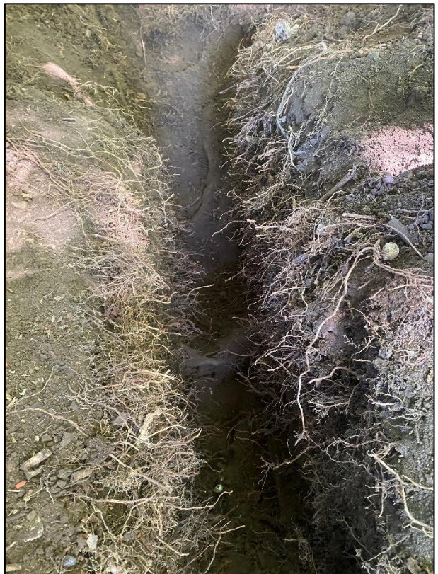
Photographs 10-13: Exploratory excavation within the CRZs of #989 & 990 encountered a cluster of medium-sized roots (~5-9cm Ø) at ~0.5m north of the proposed "Building C" corner ( above ) and a similar cluster at ~1m east of the corner ( below ). 1x ~8cm Ø and 1x ~6cm Ø were also encountered at the corner itself ( above ). An additional 1x ~6cm Ø root was encountered at ~1.5m north of the corner ( below ).
