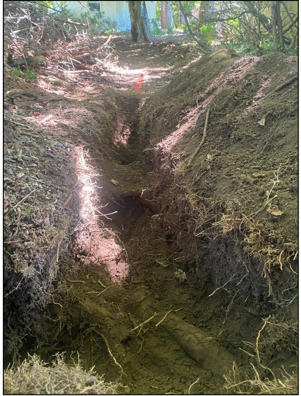
Photographs 10-13: Exploratory excavation within the CRZs of #989 & 990 encountered a cluster of medium-sized roots (~5-9cm Ø) at ~0.5m north of the proposed "Building C" corner ( above ) and a similar cluster at ~1m east of the corner ( below ). 1x ~8cm Ø and 1x ~6cm Ø were also encountered at the corner itself ( above ). An additional 1x ~6cm Ø root was encountered at ~1.5m north of the corner ( below ).
