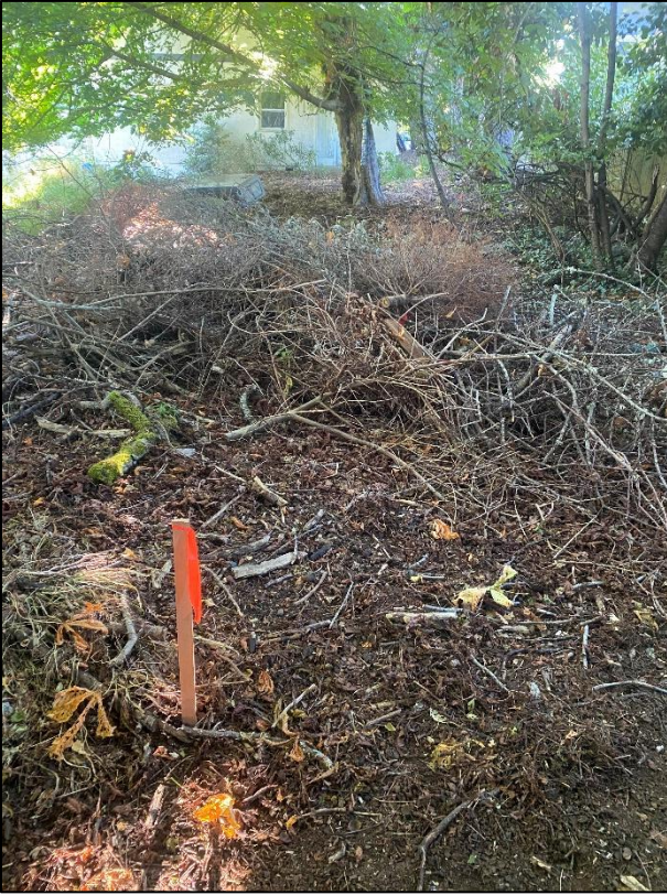
Photographs 2-5: Prior to breaking ground, the proposed corners of "Building C" were identified by a survey team using wooden stakes with orange marking ribbon. We then removed existing debris near the subject trees and delineated the lines of our exploratory excavations with orange marking paint.
