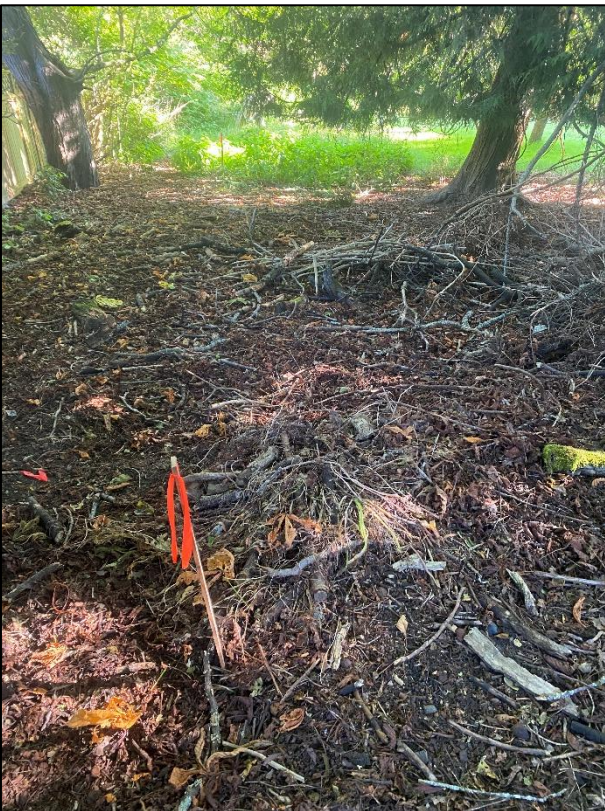
Photographs 2-5: Prior to breaking ground, the proposed corners of "Building C" were identified by a survey team using wooden stakes with orange marking ribbon. We then removed existing debris near the subject trees and delineated the lines of our exploratory excavations with orange marking paint.
