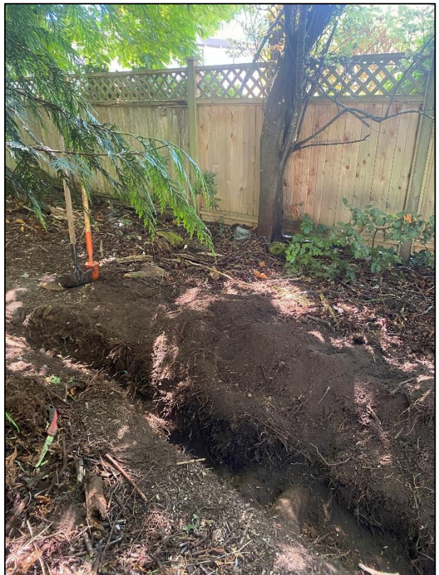
Photographs 6-9: Exploratory excavation within the CRZ of #987 encountered 1x >10cm Ø root at ~30cm south of the proposed "Building C" corner ( above ), 1x >10cm Ø root at ~4m south of the corner ( below ), a cluster of roots <5cm Ø and 1x 4cm Ø root ( upper and lower left ) at ~2-3m from the corner.
