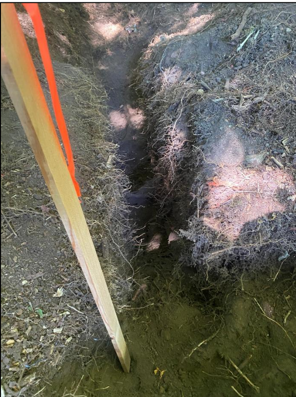
Photographs 10-13: Exploratory excavation within the CRZs of #989 & 990 encountered a cluster of medium-sized roots (~5-9cm Ø) at ~0.5m north of the proposed "Building C" corner ( above ) and a similar cluster at ~1m east of the corner ( below ). 1x ~8cm Ø and 1x ~6cm Ø were also encountered at the corner itself ( above ). An additional 1x ~6cm Ø root was encountered at ~1.5m north of the corner ( below ).
