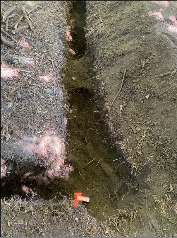
Photographs 10-13: Exploratory excavation within the CRZs of #989 & 990 encountered a cluster of medium-sized roots (~5-9cm Ø) at ~0.5m north of the proposed "Building C" corner ( above ) and a similar cluster at ~1m east of the corner ( below ). 1x ~8cm Ø and 1x ~6cm Ø were also encountered at the corner itself ( above ). An additional 1x ~6cm Ø root was encountered at ~1.5m north of the corner ( below ).
